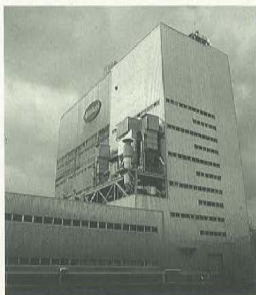
Emissions from the detergent production facility in Italy were reduced.
